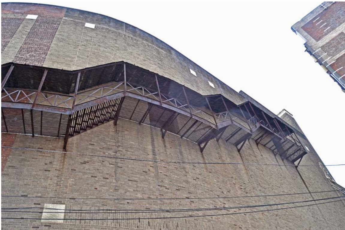
Photo 11: Loew's Jersey Theatre. 54 Journal Square, Jersey City, NJ 07306. Covered metal fire escape along south elevation. July 9, 2021.
