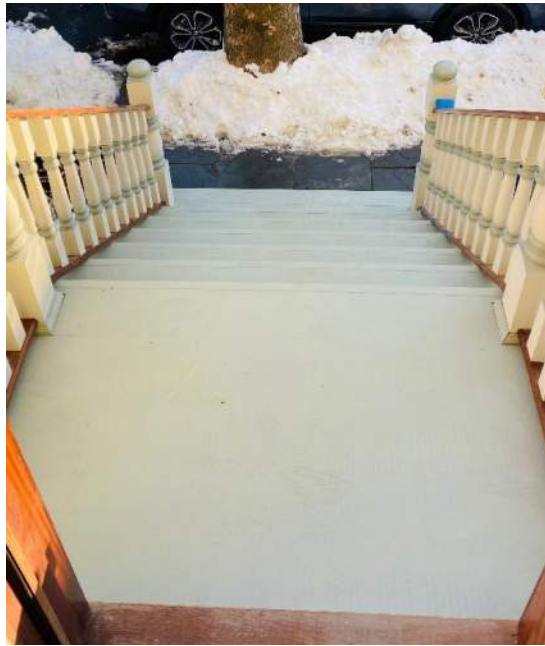
5. The stoop steps have been re-constructed in wood.
