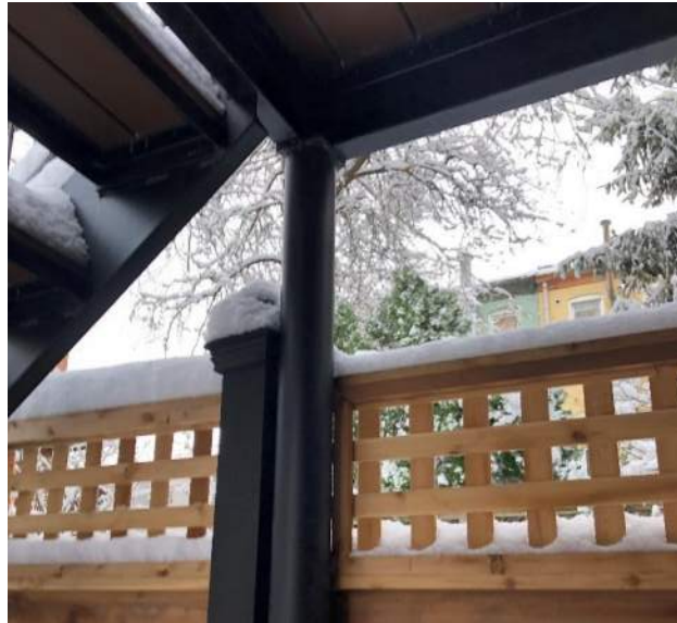
8. Photo showing structural column tucked behind fence post
