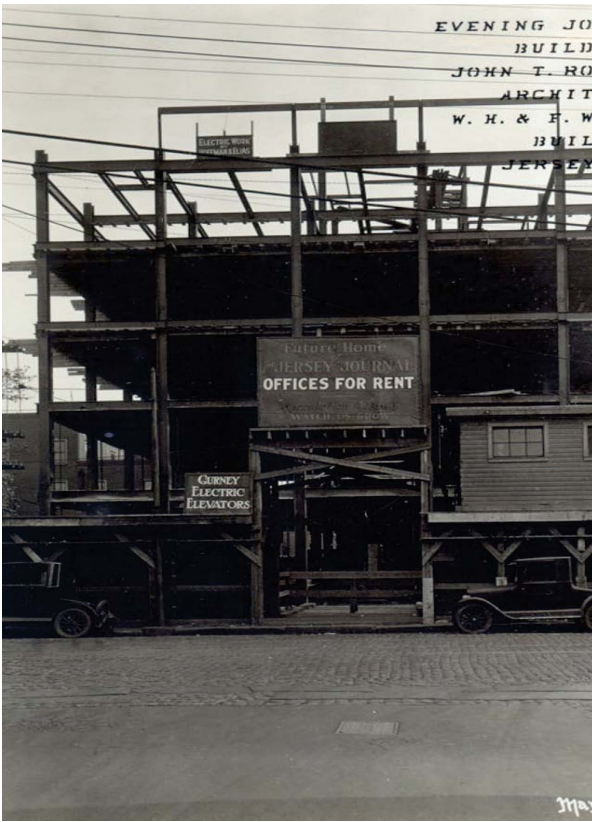
30 Journal Square Construction, 1924
