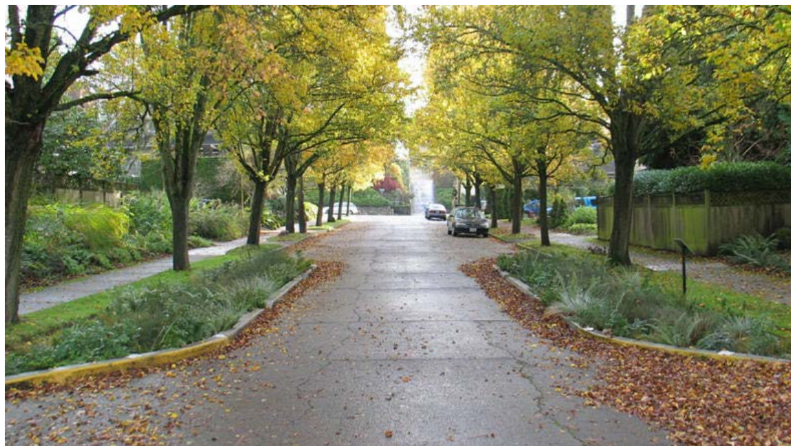
Figure 36: Street Trees and Curb Bulb Outs with Bioretention (Source: Low Impact Development Center)
