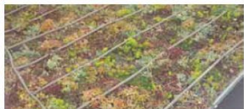
Above: Drip Irrigation lines laid on top of Eco-Standard Trays at the time of installation.
