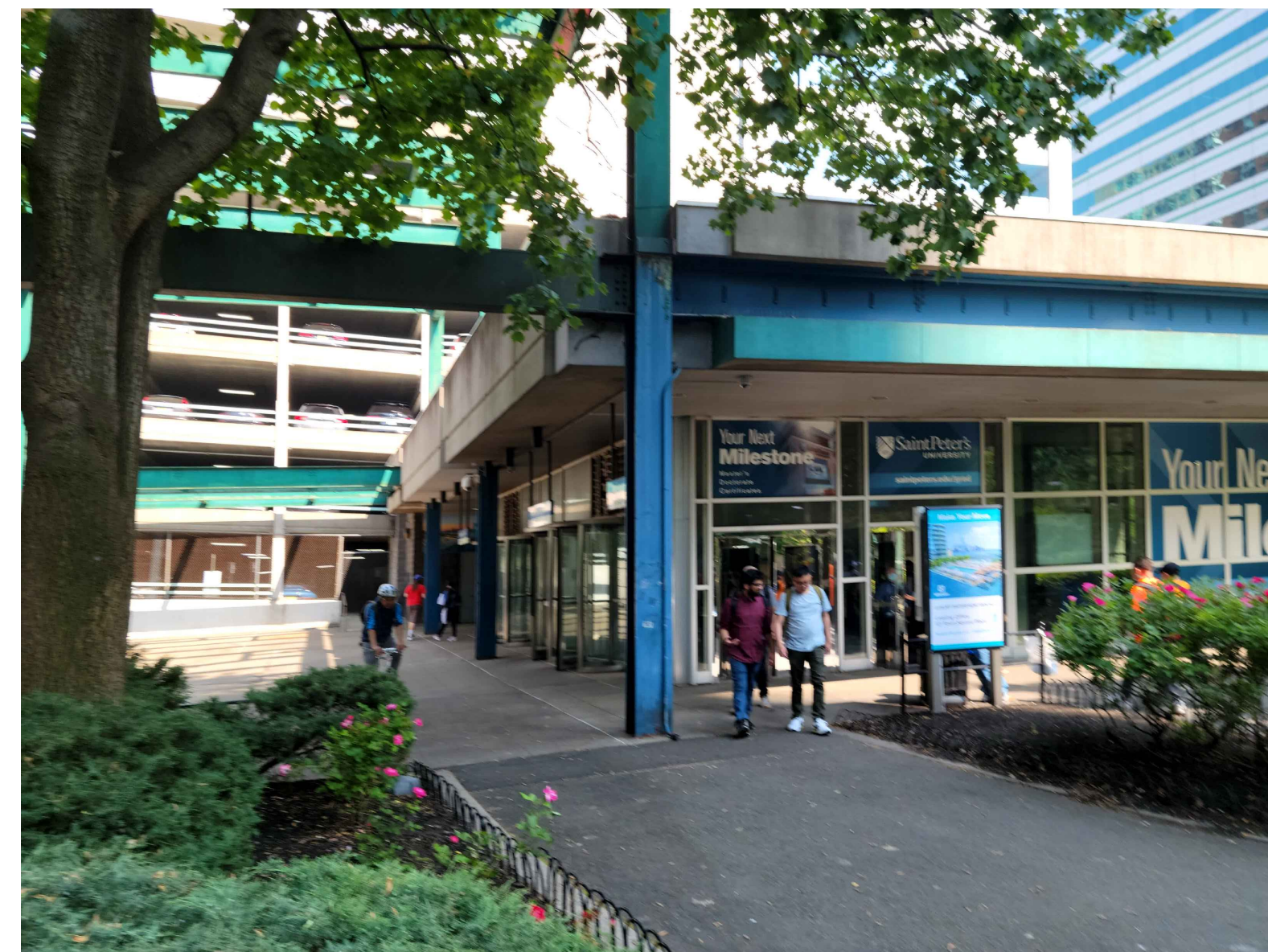
5 PATH STATION SW CORNER LOOKING NORTH
