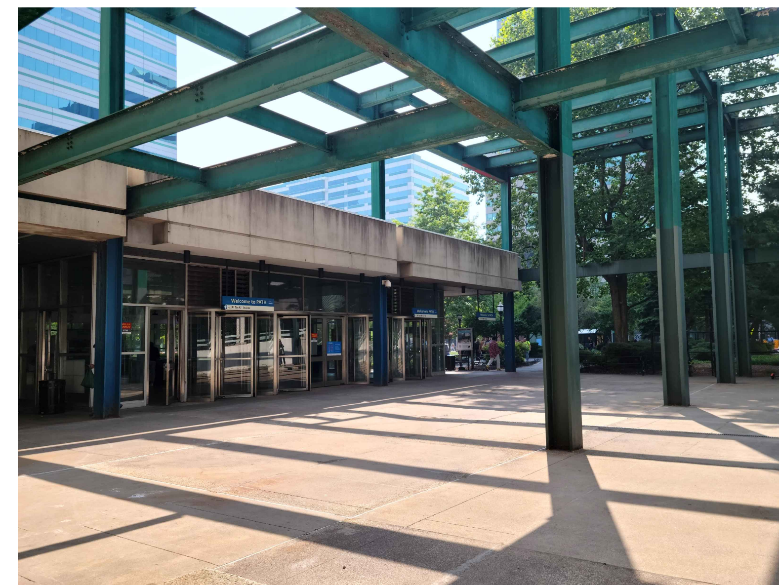
1 NW CORNER OF SITE LOOKING SOUTH EAST
