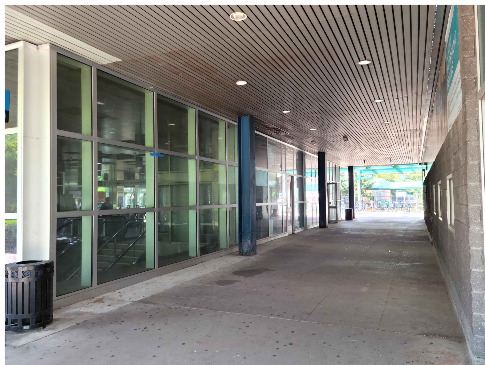
7 PATH STATION EAST SIDE LOOKING NORTH
