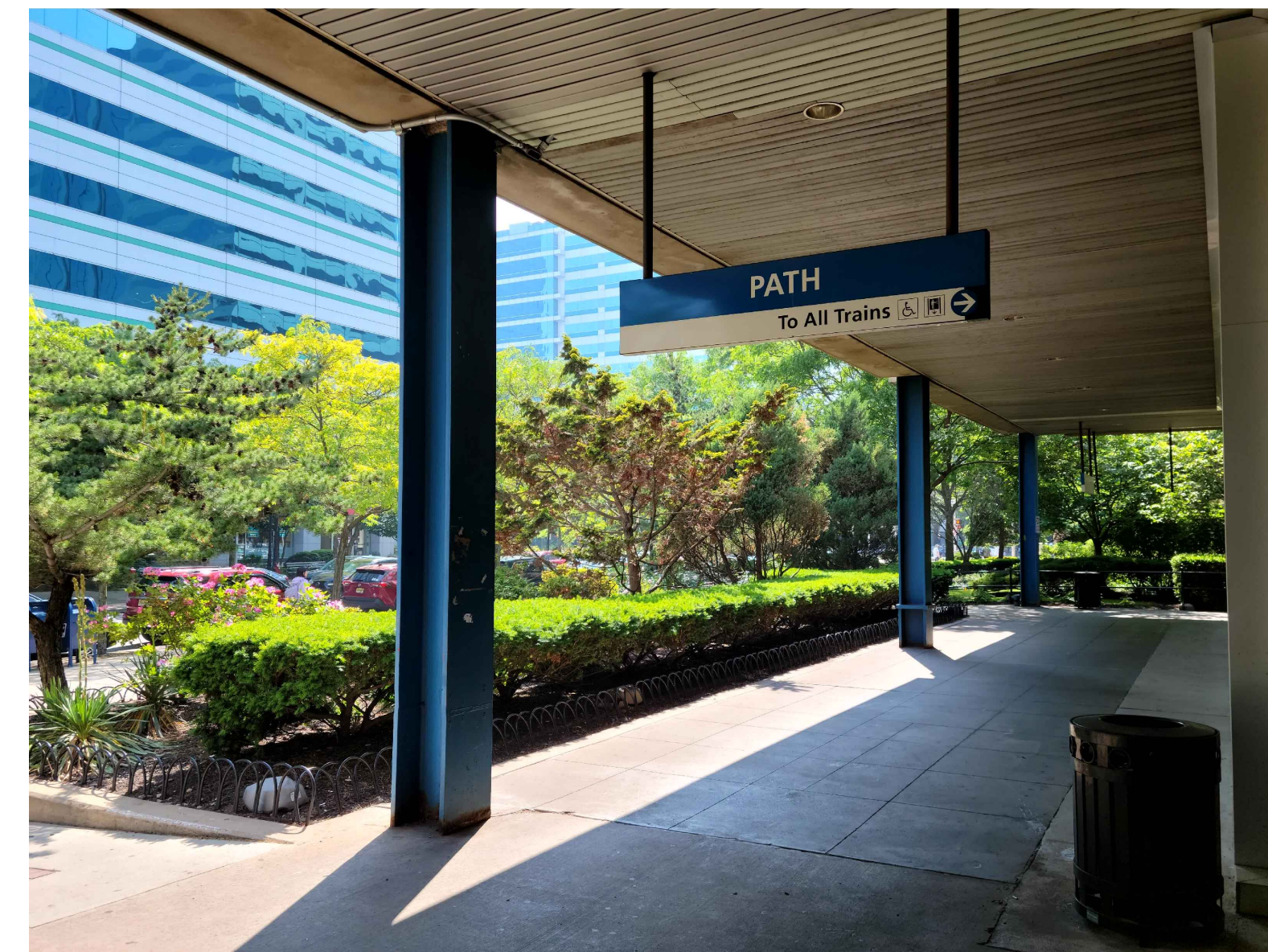
2 PATH STATION SOUTH SIDE LOOKING EAST
