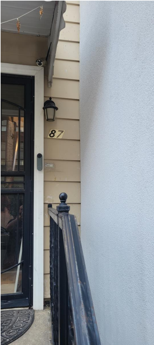
Photo 1-1: Front house view with connection to 87/89 Monitor
