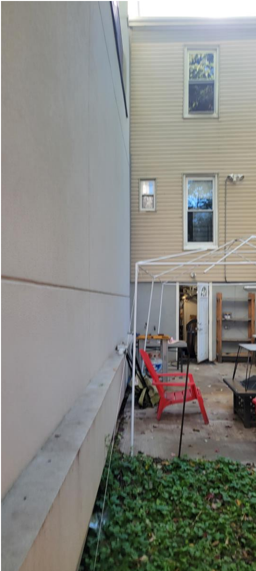
Photo 1-3: Rear view with connection with 87/89 Monitor
