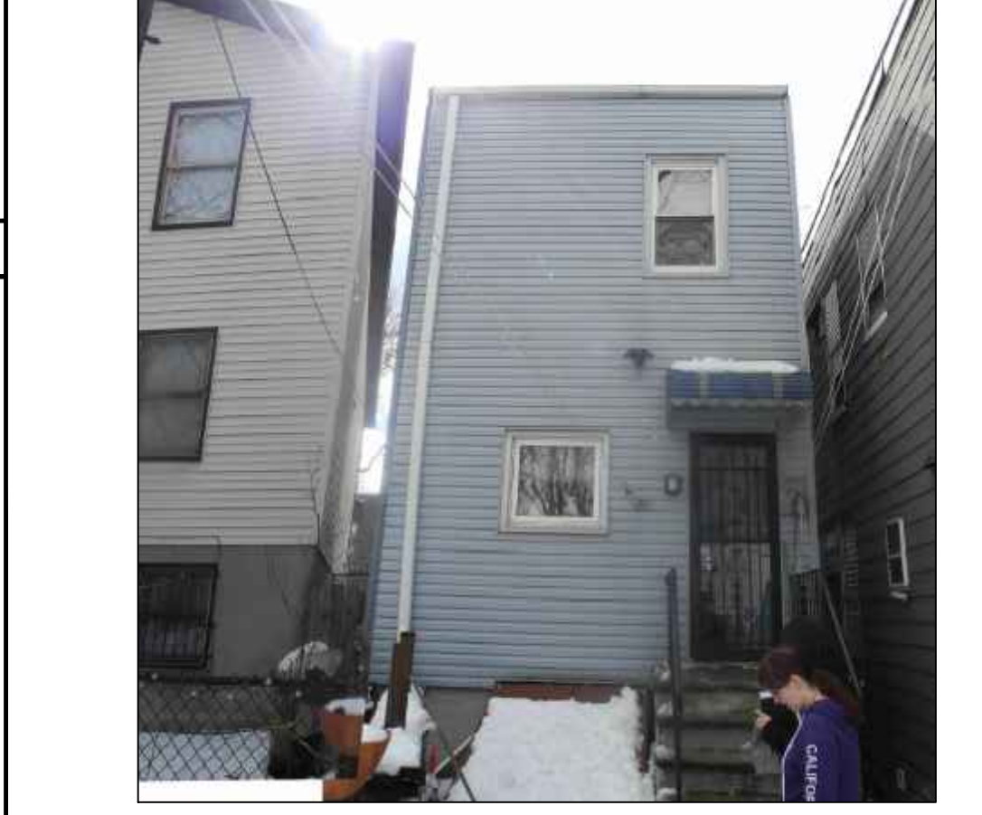
4 BACK VIEW OF EXISTING HOUSE
