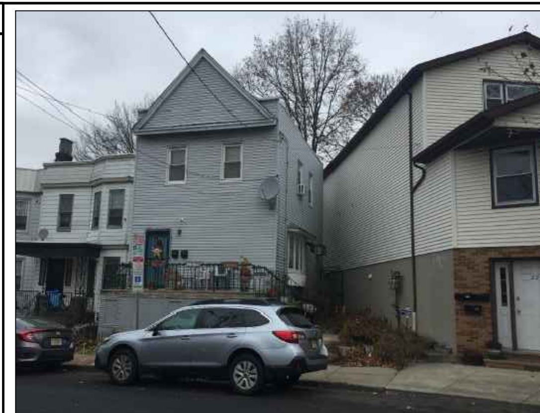
3 FRONT VIEW OF EXISTING HOUSE
